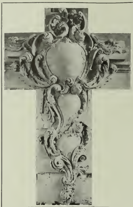
DETAIL BY TOLEDANO & WOGAN, ARCHITECTS. Executed by the Northwestern Terra Cotta Company.
